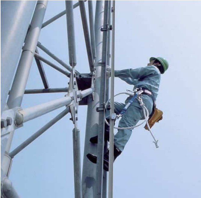
FM Skylock installed on the transmission tower.
