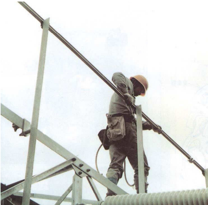
Fuji Lock installed on the outdoor iron structure.
