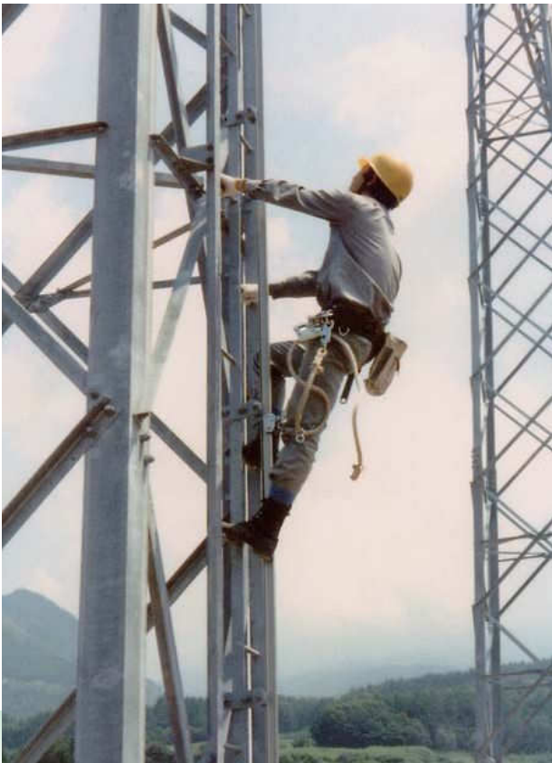
FM Skylock installed on the transmission tower.
